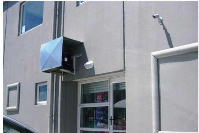
EXAMPLE OF CCTV AT REAR OF PREMISES
