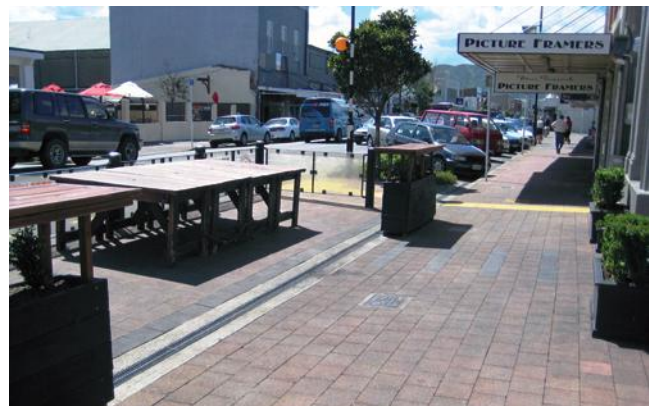
EXAMPLE OF POOR DEMARCATION OF OUTDOOR DRINKING AREA
