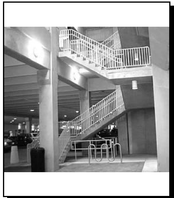
This open stair provides good visibility from store entrance as well as the parking area.
