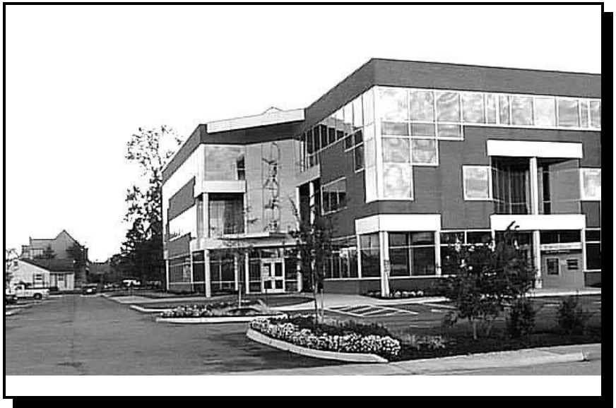
A well maintained office building with good visibility around the entire perimeter.
