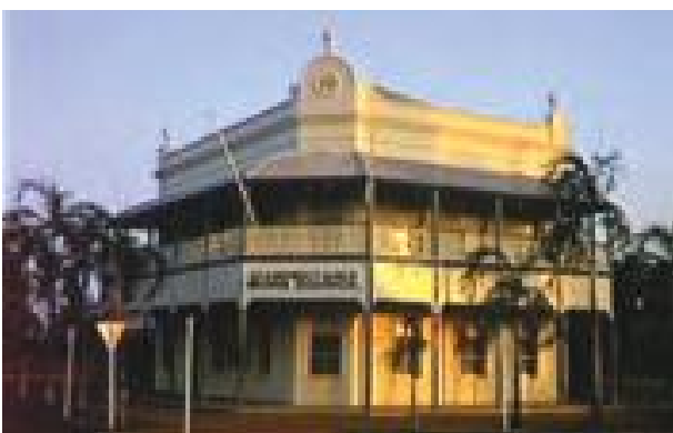
Landmark buildings as key parts of centres
