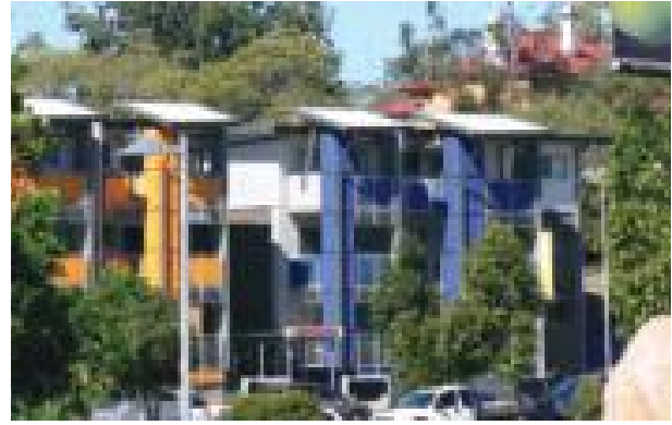
Affordable apartments in the suburbs
