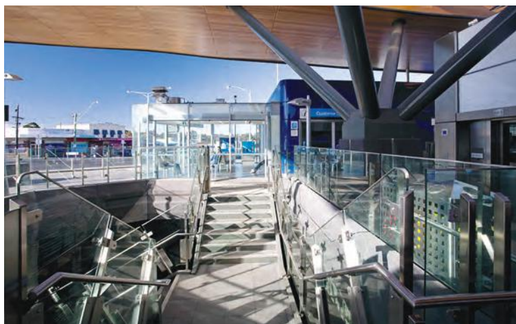
Figure 2.7: An example of recent station design in Nunawading, Melbourne
