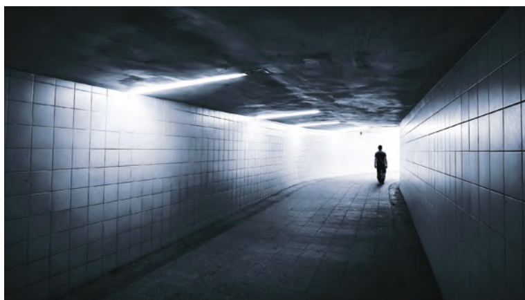
Figure 2.1 (a): Underpasses are not only inherently dangerous places. A lack of maintenance and repair can also create vulnerable settings
