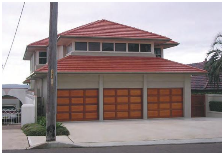
Figure 2.4: This house does not sufficiently balance territoriality with opportunities for surveillance of the street
