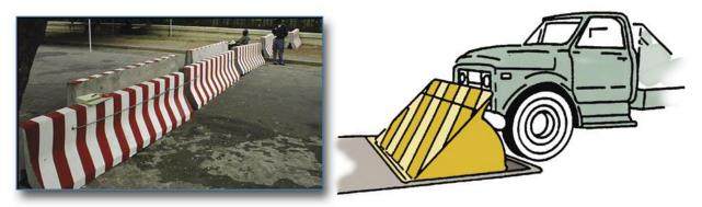
Figure 2-14 Examples of active and passive vehicle barriers
