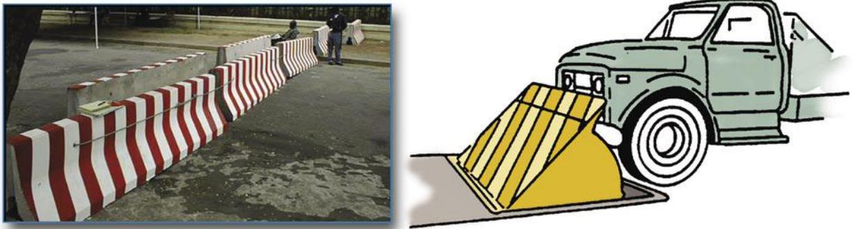
Figure 2-14 Examples of active and passive vehicle barriers
