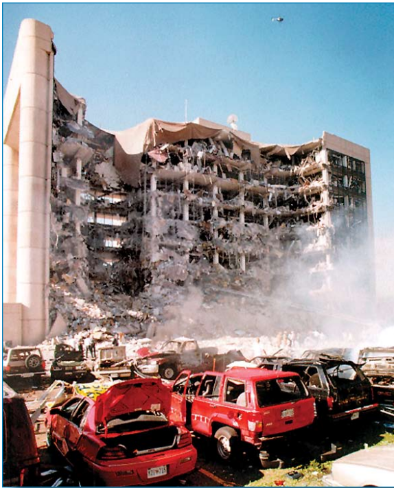
Figure 2-4 Alfred P. Murrah Federal Office Building
