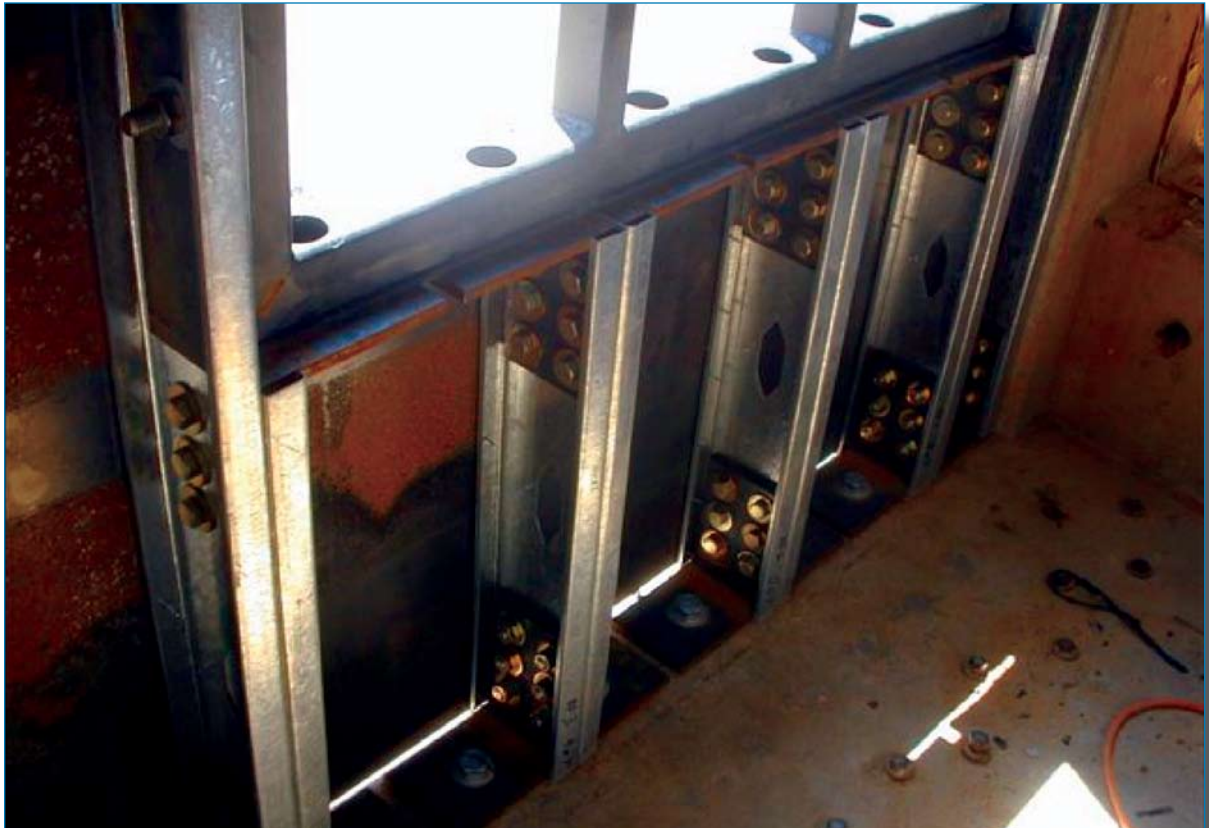
Figure 2-19 Metal stud blast wall
