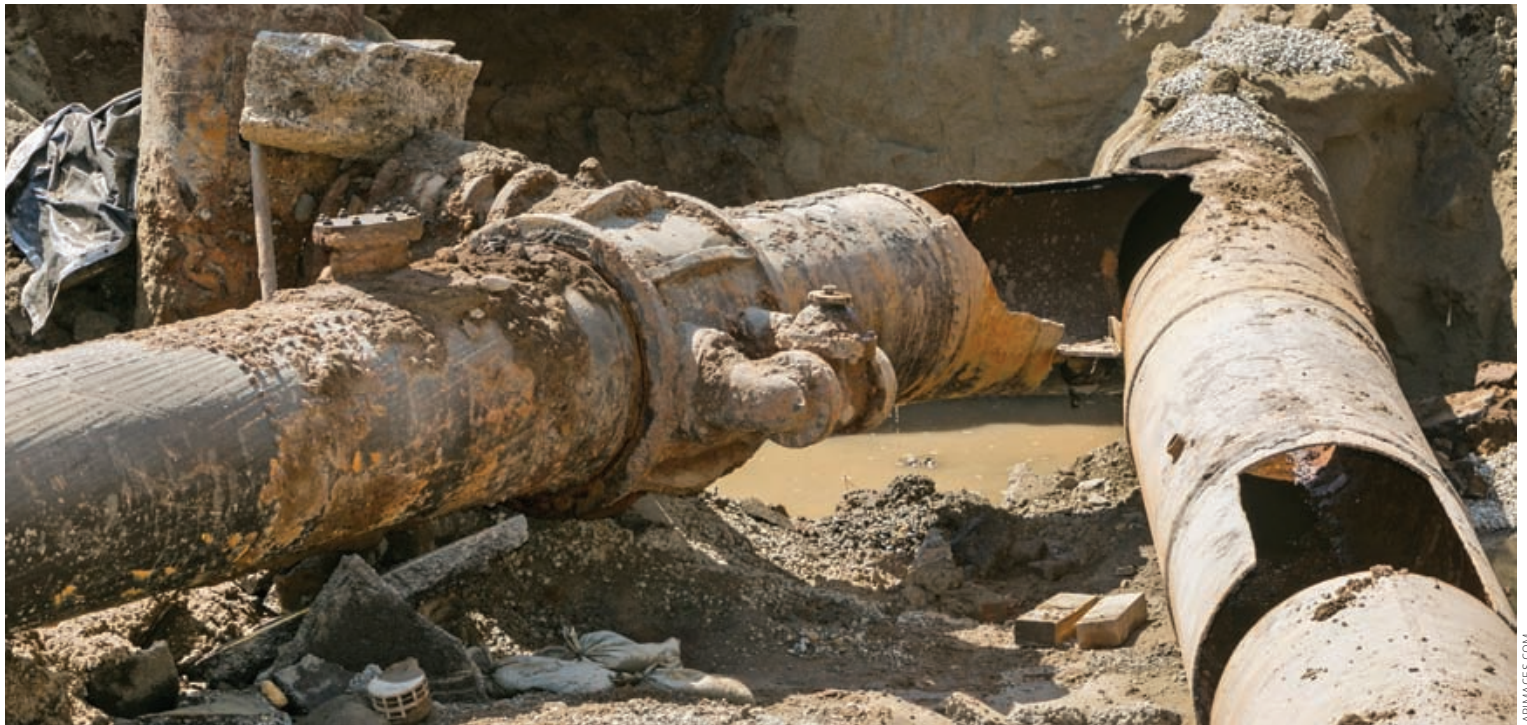
A “Y”-shaped juncture connecting two main trunk lines that ruptured is seen on Sunset Boulevard in Los Angeles after the 1994 Northridge earthquake. Mayor Eric Garcetti’s call to strengthen Los Angeles’ water system — a pillar of his plan to ready the city for a major earthquake — would cost up to $15 billion and require decades of work.
