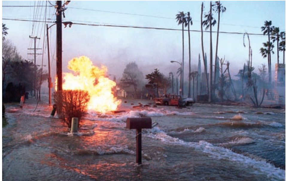
Gas from a ruptured supply line burns as water from a broken water main floods Balboa Boulevard in the Granada Hills area of Los Angeles after the predawn Northridge earthquake struck in 1994. A lack of water would be the biggest disruption to area businesses during the Big One.
